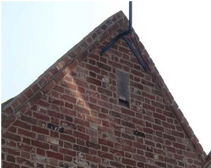
Bat tube integrated within building fabric (ref: Schwegler Natur)
