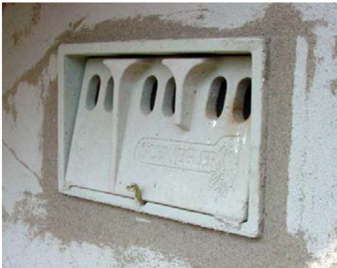
Sparrow terrace integrated within brick / concrete walls (ref: Schwegler Natur)
