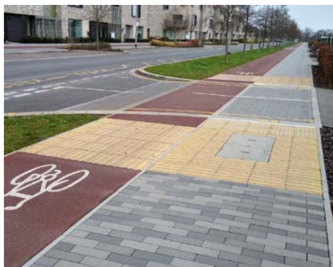
Tactile pavement used at junction of segregated cycle/footpath and road
